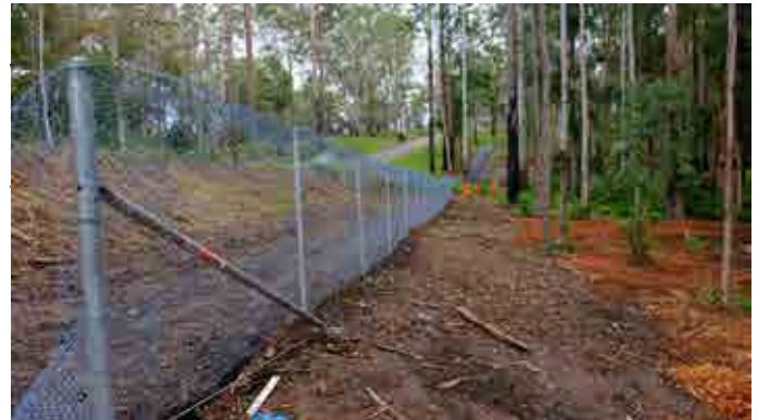
Photo: W. Ashwood – newly erected fence around the periphery of the project site to prevent wildlife entering or koalas leaving.
